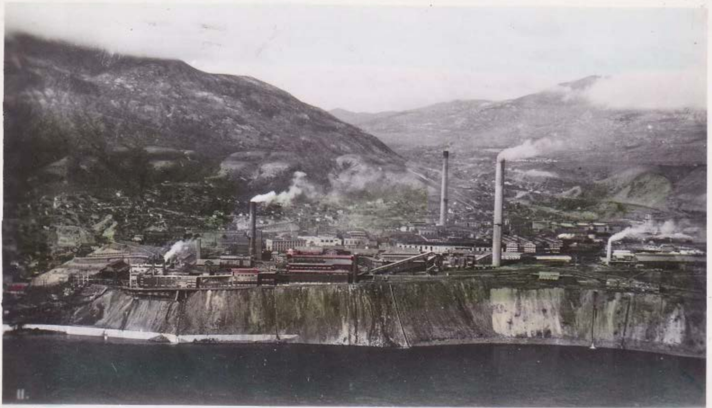
TRAIL SMELTER FROM EAST TRAIL, B.C.
